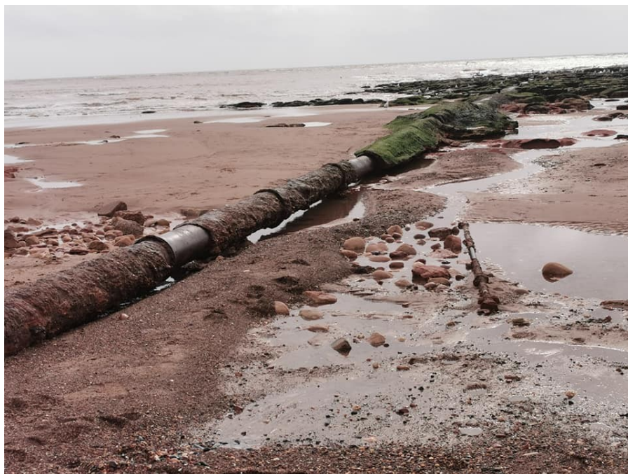
Pipe from the CSO storage tank on the Maer
